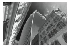
Waviness is calculated by quantifying distortion in a reflected image.
